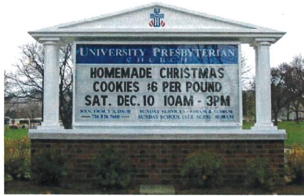
Figure 9-3: Illustration of a sign for an institutional use on a brick base with foundation plantings.
